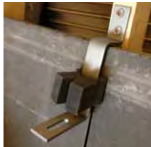
Step 2: Put SolarFlash (small) on the bracket.
