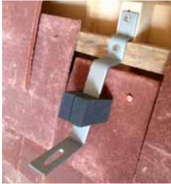
Step 1: Fix foam to the bracket drop.
