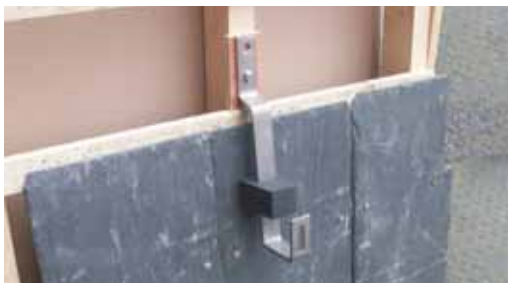
Step 1: Fix foam to bracket drop.
