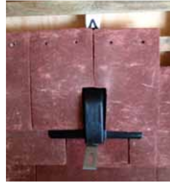
Step 3: Cut tiles around the hood of the SolarFlash as per page 10.
